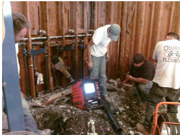
The men's room under reconstruction.
